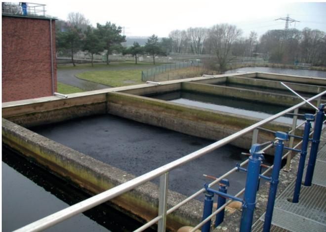
Figure 3: Open GAC-filter at the wastewater treatment plant Obere Lutter (Source: AOL)
